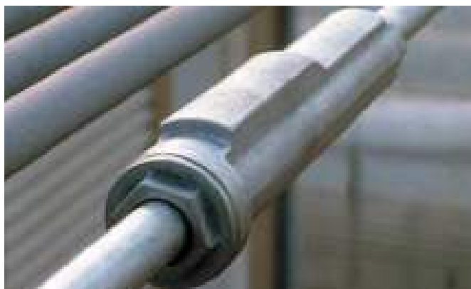
Figure 14A: Expansion fitting.
