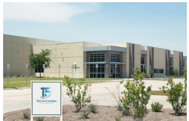
T5@Dallas, the state-of-the-art data center in Texas.
