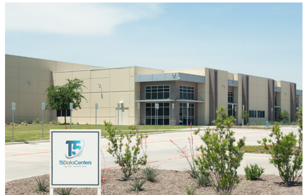
T5@Dallas, the state-of-the-art data center in Texas.
