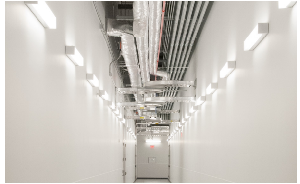
20' EMT installs twice as fast as 10' conduit.
