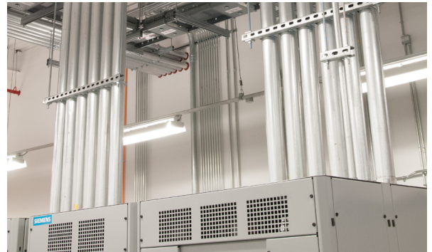
20' EMT installs straight for easy equipment hookups.
