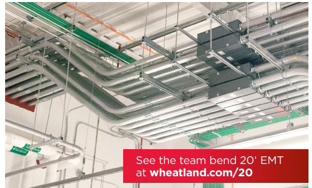
20' EMT bends easily around existing MEP systems.
