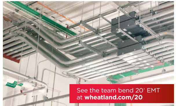
20' EMT bends easily around existing MEP systems.
