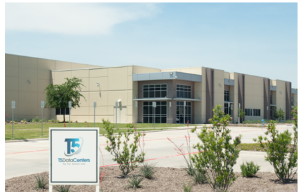
T5@Dallas, the state-of-the-art data center in Texas.
