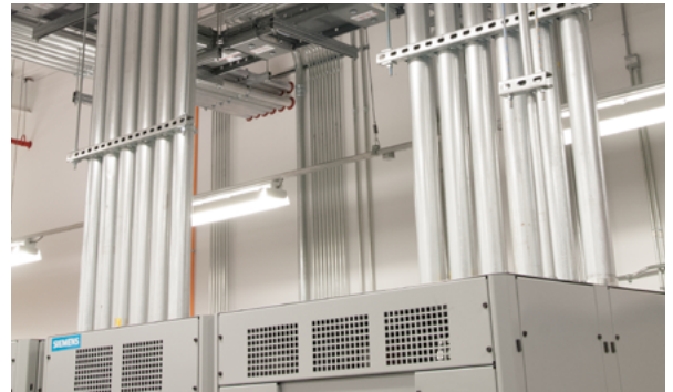
20' EMT installs straight for easy equipment hookups.
